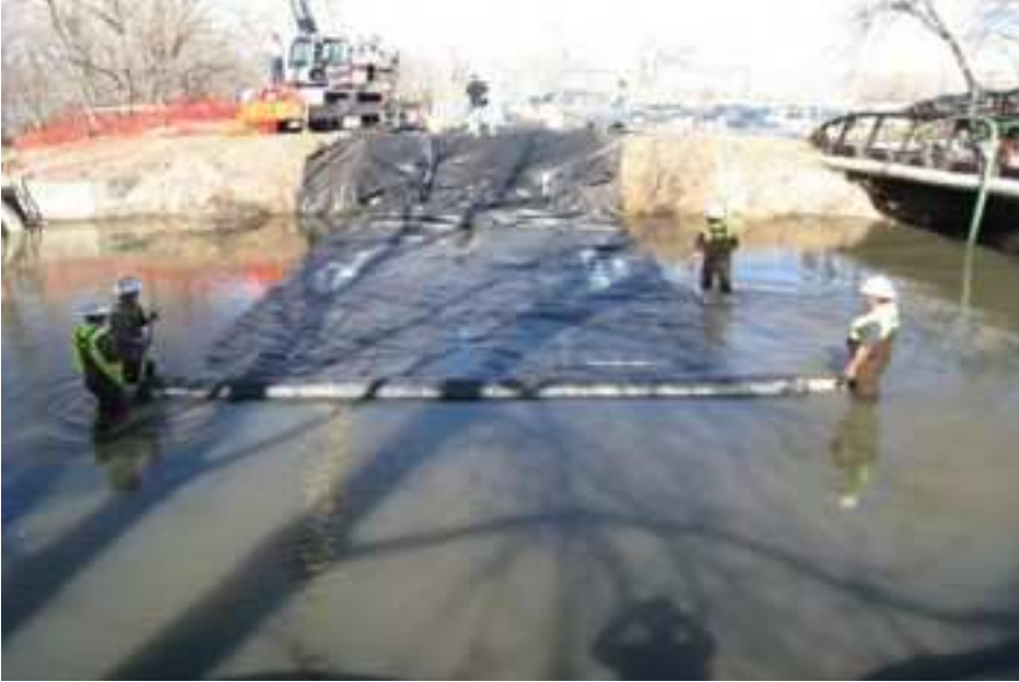
A Dam-It Dams Cofferdam unrolling as it fills with water
