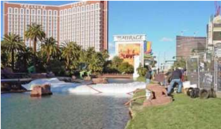
A Dam-It Dams Cofferdam creating a water barrier
